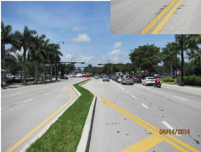
Hillsboro Boulevard East of Federal Hwy looking West
