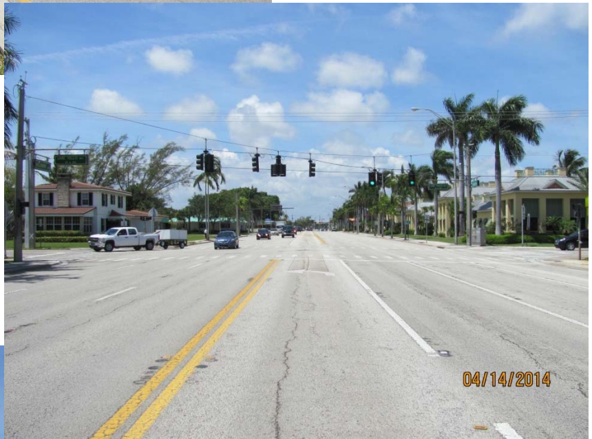
Hillsboro Boulevard East of NE/SE 6 th Ave looking West
